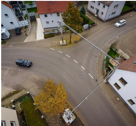
Photo of the test junction. Source: UULM-MRM
