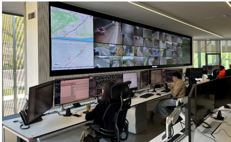
Autopistas Operations and Road Safety Centre
